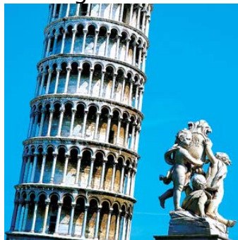
Leaning Tower of Pisa
